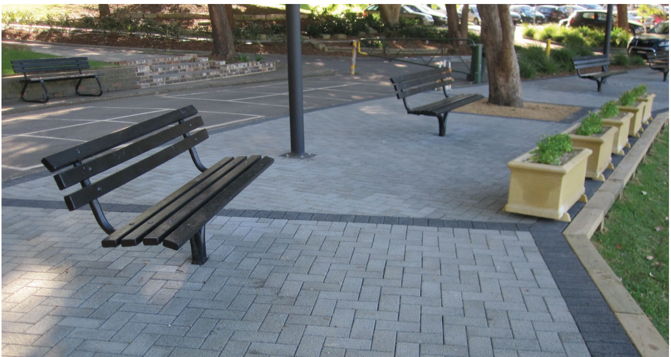
Permeable paving in nature strip – provides water infiltration to street tree root systems and reduces surface runoff (Photograph: HydroCon Australasia hydroston.com.au)
