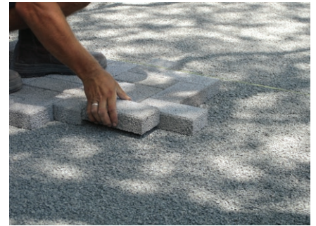
Laying permeable paving (Photograph: HydroCon Australasia hydroston.com.au)
