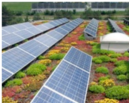
Solar panels have improved efficiency when used in combination with green roofs
